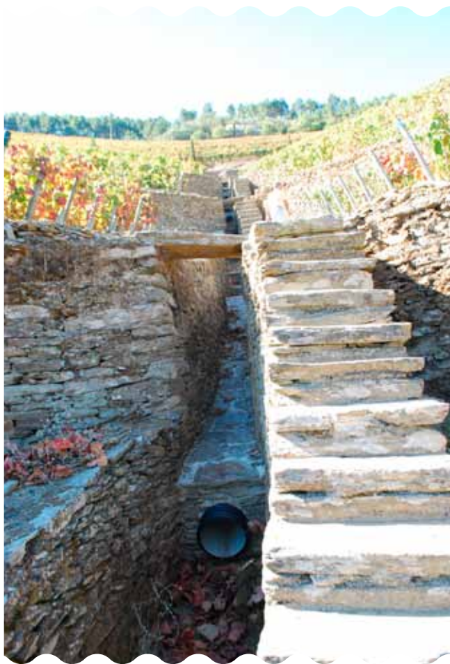
FIGURES 8A AND 8B - On the left, a correct drainage system along a water course dating back to pre-phylloxera times; on the right, the same system after it was destroyed upstream to make way for mechanized patamares, resulting in serious erosion to the embankments.
