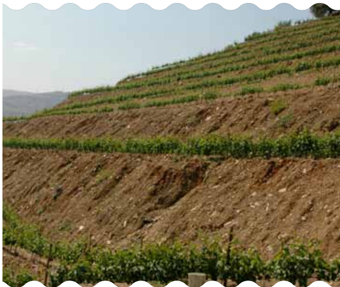
FIGURE 4 - High, steeply-sloped embankments scarred by multiple furrows created by surface water due to the lack of an effective system for preventing erosion.
