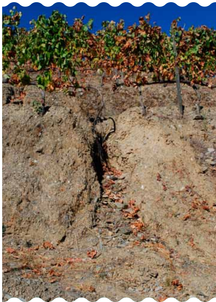
FIGURES 15A AND 15B - Narrow patamares whose horizontal surfaces are occasionally responsible for erosion to the embankments because there are no drains to carry the surface water down the length of the terrace.
