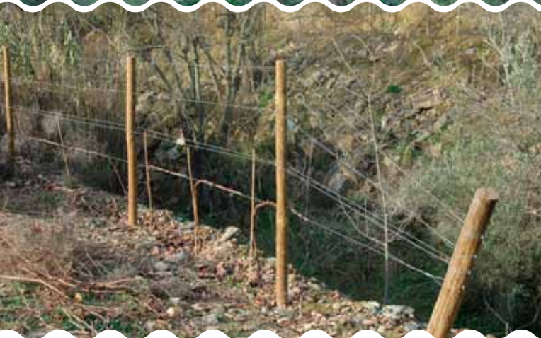
FIGURES 25A AND 25B - Methods of anchoring an end post: Above, wood anchor with a tension wire; mobile wires with a turnbuckle; below, 2m-long anchor buried at 0.8-1.0m to reduce the strain on the end post and make it easier to move the double wires.
